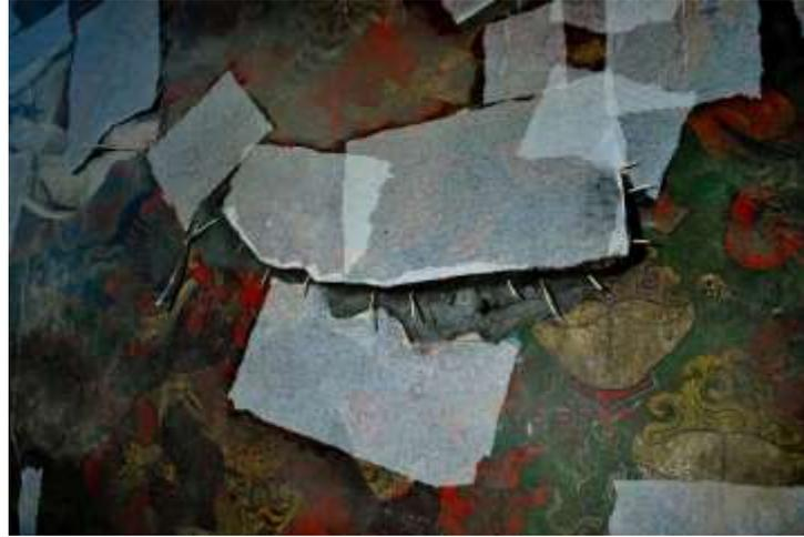
**Fig. 15** The north wall in the main hall; the edges have been filled with new earthen plaster and bamboo sticks inserted into gaps (courtesy of K.P.)
