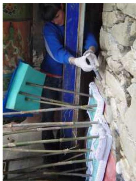
**Fig. 16** Klara injecting prepared grouting between the wall paintings and the stonework, on the west wall in the porch
