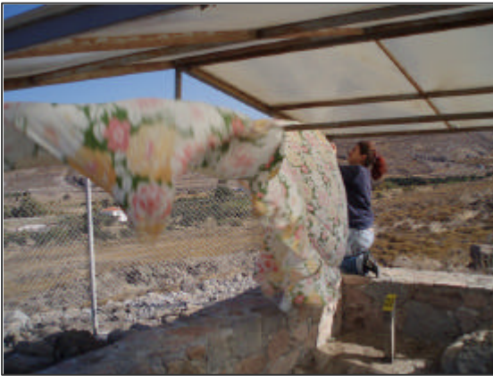
Fig.8 – Evangelia Kyriazi installing sheets on site to give us shelter from the wind.
