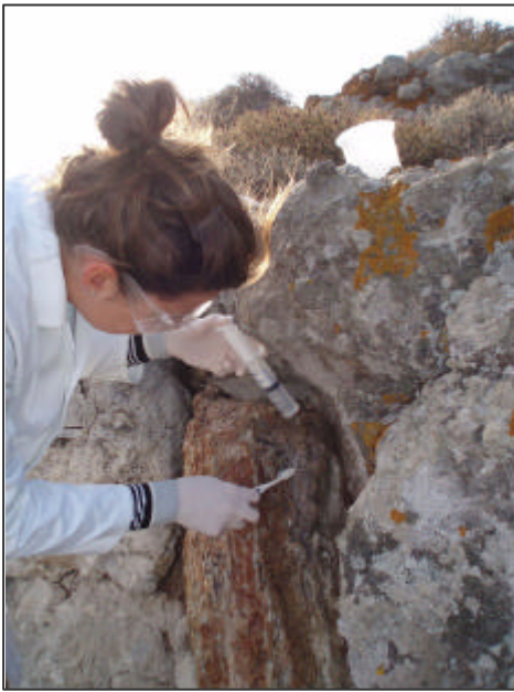
Fig.9 – Removal of lichen and biological growth with hydrogen peroxide 50%.
