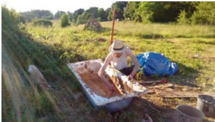
Figure 20. Preparing our first layer of plaster: the slurry
