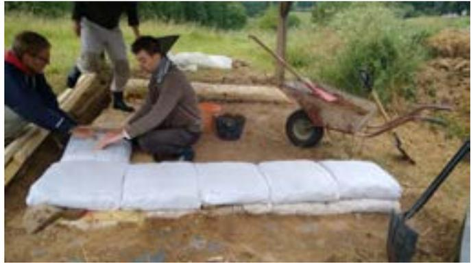
Align the earth-bags in such a way that they form perfectly straight vertical walls. This step is crucial in order to secure the proceeding straw bale walls in place.
