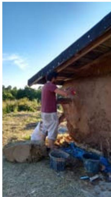
Figure 22. Application of third layer of plaster (1:1 clay:sand)
