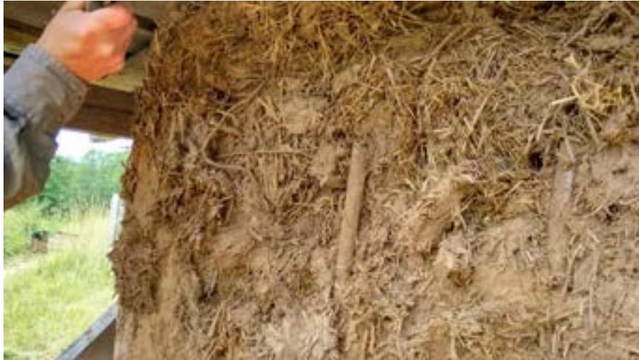
Figure 10. Wooden pegs and sticks are used to compress straw bale walls
