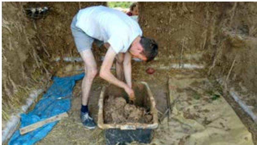
Figure 21. Preparation of cob plaster
