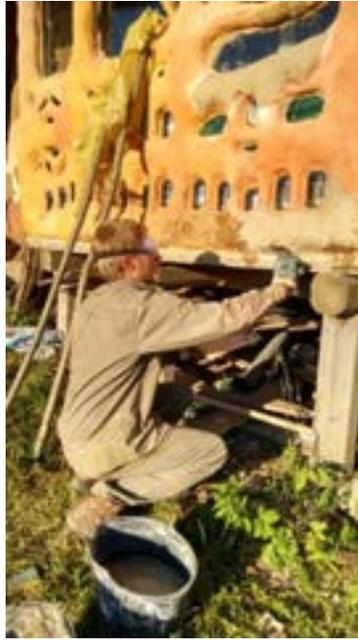
Figure 24. Application of lime plaster
