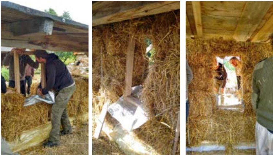
Figure 16. Installing window frames and damp-proofing windowsills
