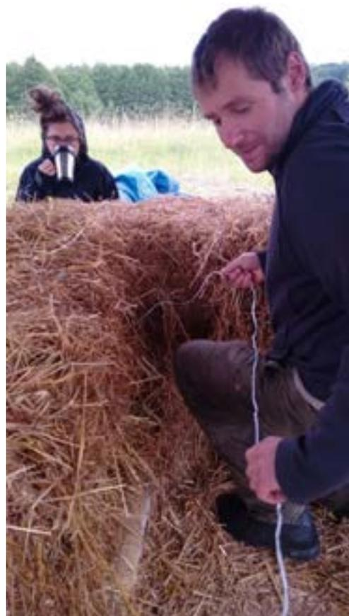
Figure 14. Compression using straw bale needle and string
