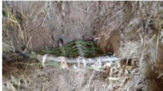
Figure 23. Wattle and daub method involves twining sticks horizontally and vertically to create a frame/wall over which plaster is applied.
