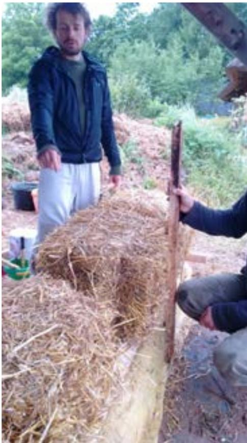
Figure 13. Using a wooden plan to assure that the layers of straw bales are perfectly aligned
