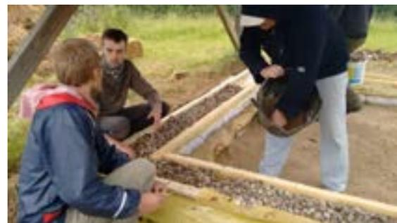
Insulate the foundation wall using wooden frames and pebbles
