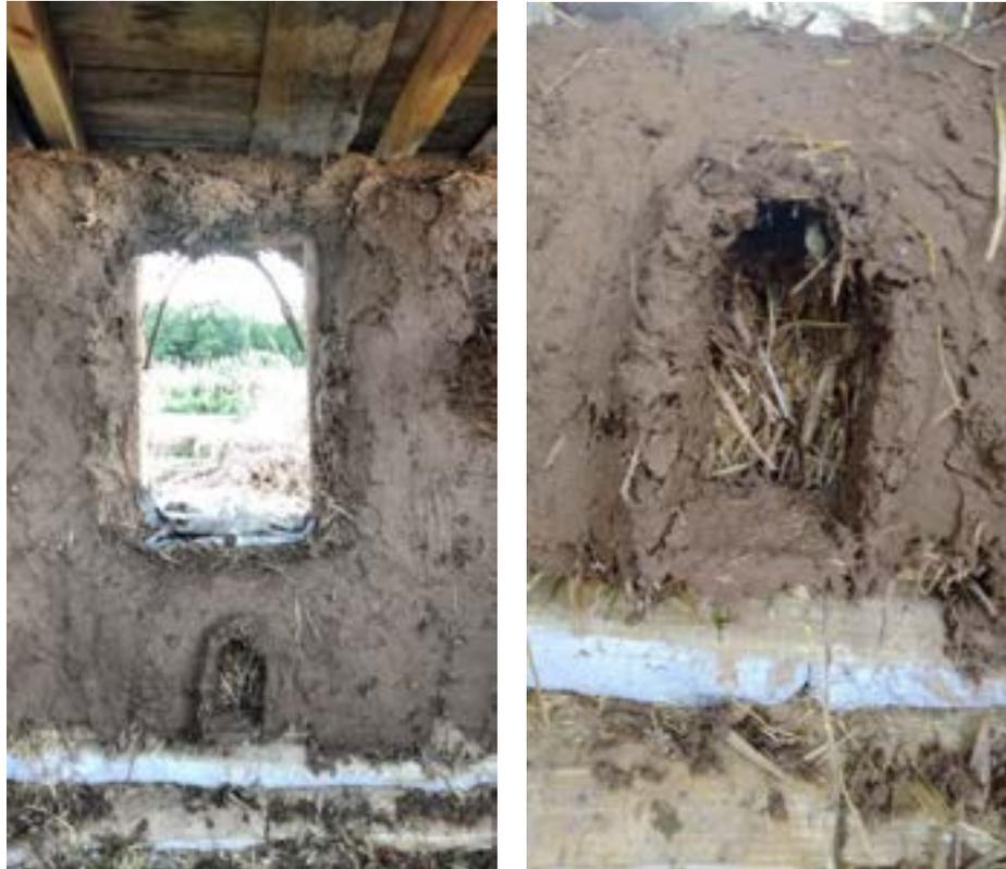
Figure 19. Making a ‘True Window’ when plastering straw bale walls
