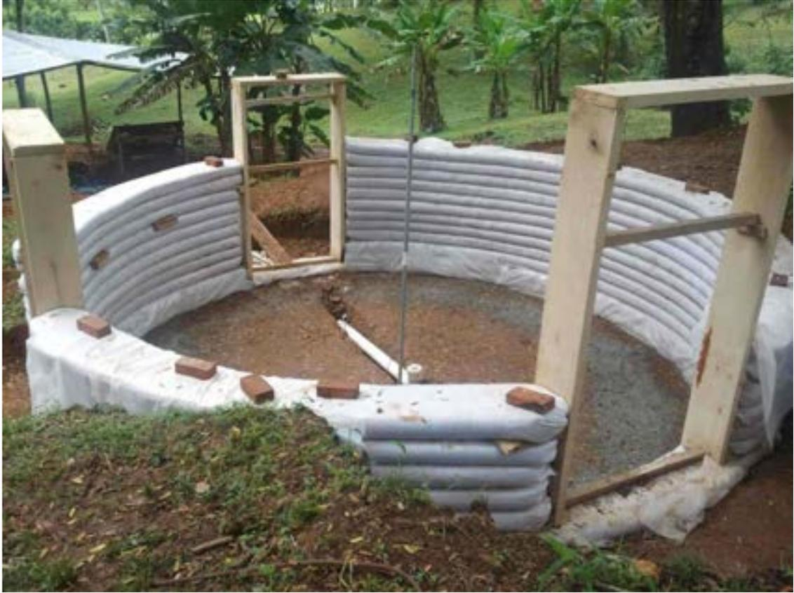
Figure 11. An example of earth-bag construction in process
