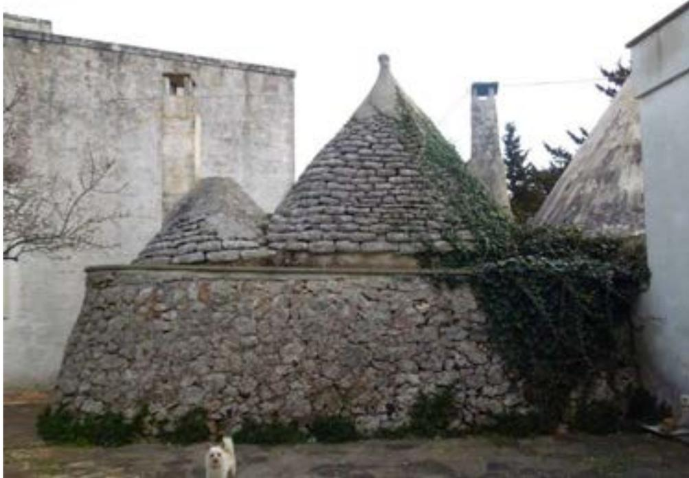
The trullo before its repair. The chianche had started to slip and vegetation had disturbed the stonework. As a result water had started to ingress and the damage needed halting.
