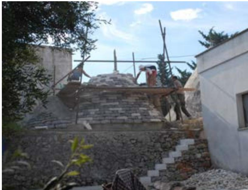
Addition of scaffolding to reach the final courses. On the right the newly installed stairs improving access to the roof.
