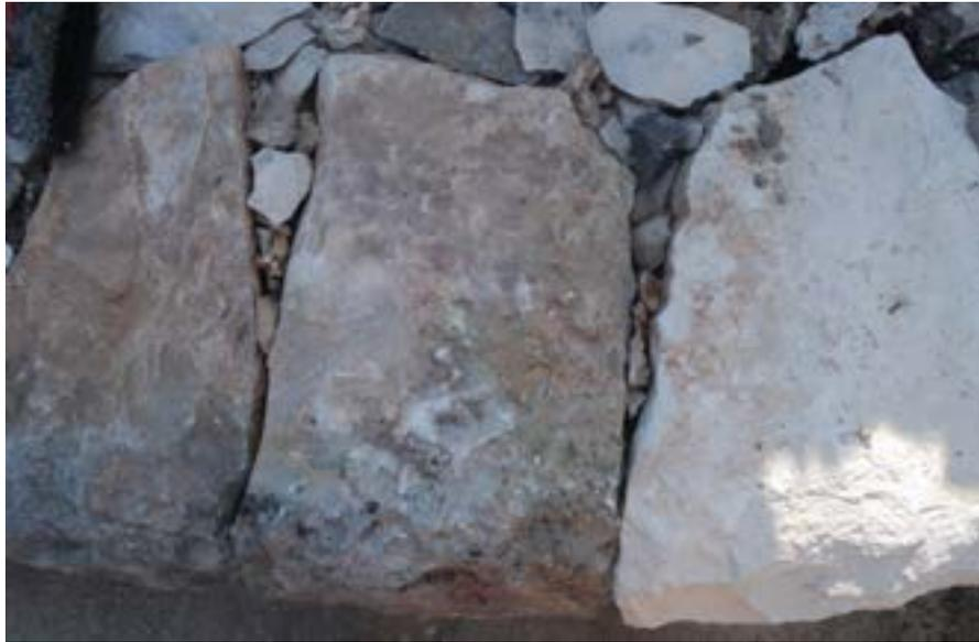
Tightly fitting chianche packed with hearting to strengthen the structure.
