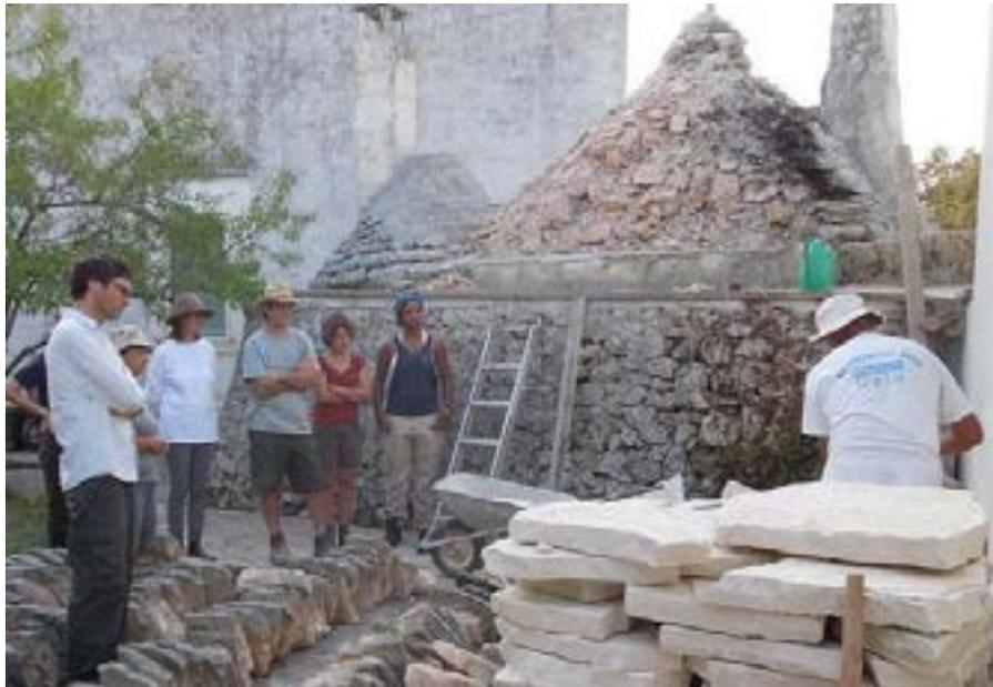
The large trullo roof on the right is without its chianche. On the floor (left) are old chianche which have been sorted into size and thicknesses. Mario is pictured on the right, behind the new limestone, showing us how to cut the large slabs.
