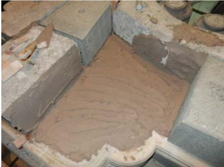
*Figure 34: The mortar bed for the stone*
