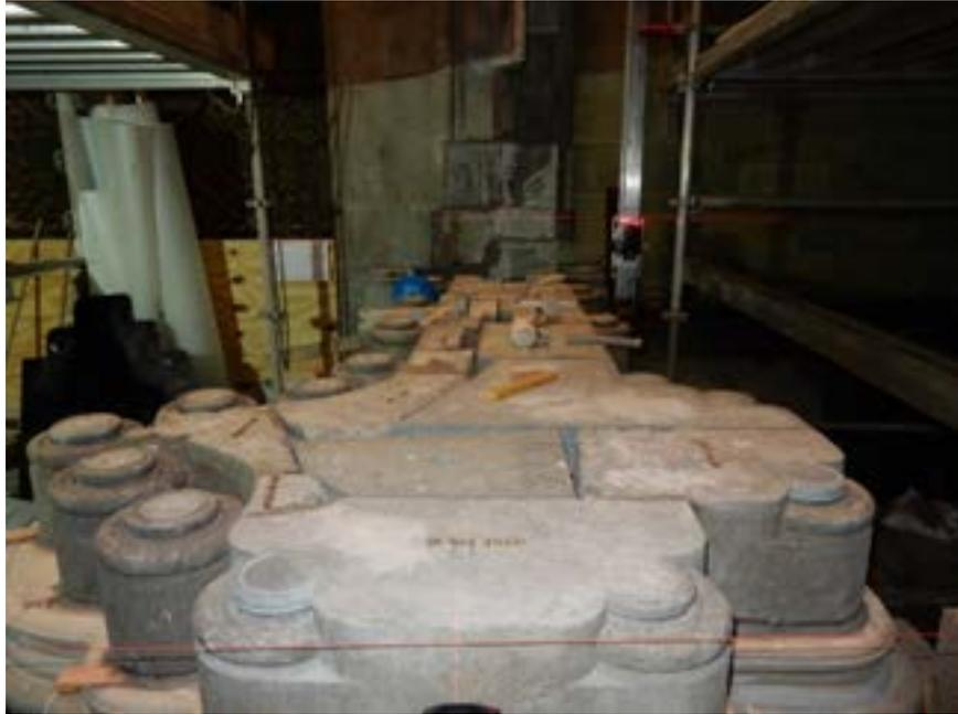
*Figure 36: Lines and laser check to ensure it is plumb and level*
