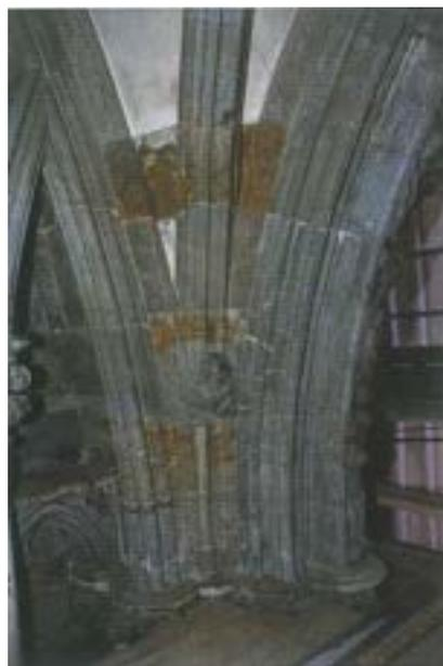
*Figure 11: Deterioration of the soapstone in situ*
