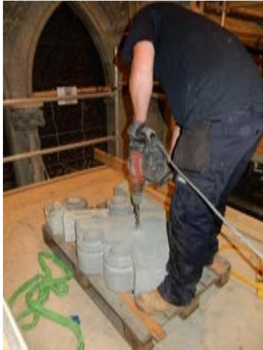
*Figure 28: Preparations for the Lewis Pins*
