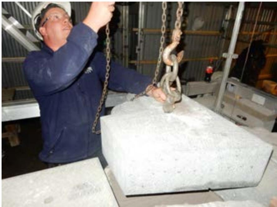
*Figure 35: Lowering the stone onto the mortar bed*
