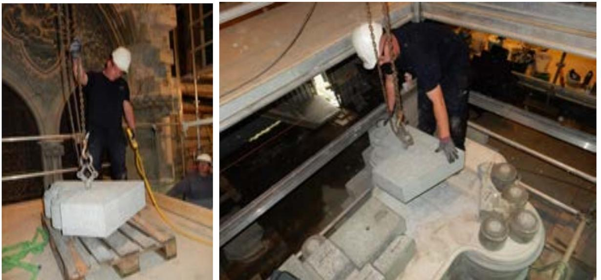
*Figure 29-29: Lifting of stones with Lewis Pins and 'dry' laying stones to check position and dimension*
