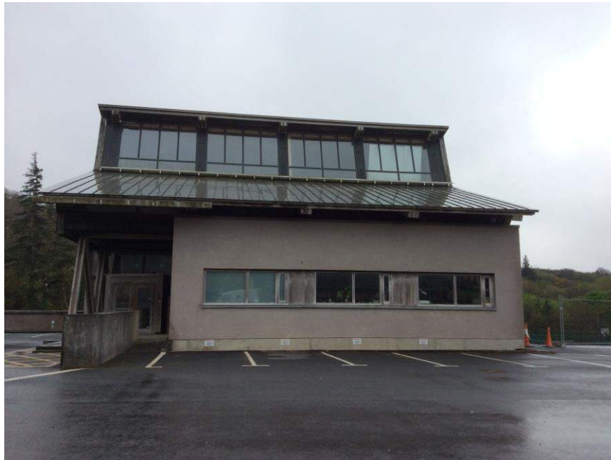
The Conservation Letterfrack workshop.
