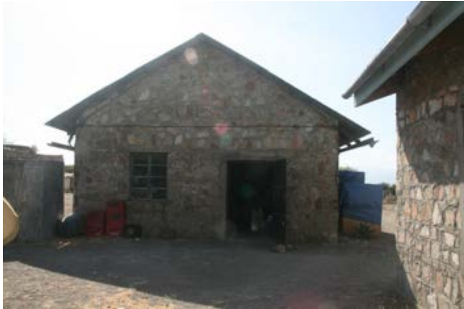
Figure 7. The Laetoli lab- our conservation lab for the season. Space was limited in this building as it was also shared by other researchers. Photograph by A. Duckor
